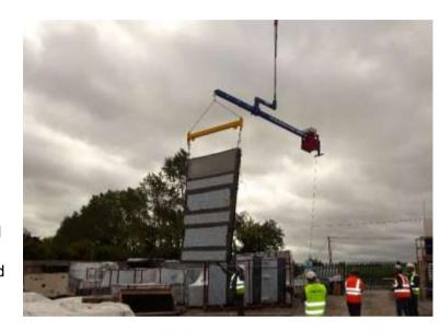
The beam has a fully rechargeable battery pack on board and also comes with two remote controls so one operator can attach he load at ground then a second operator can operate the beam for installation, so no time is lost waiting for an operator accessing the upper levels of the building.
